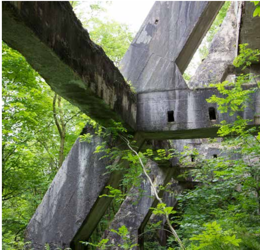
Lime kiln ruin near Buxton, Derbyshire
