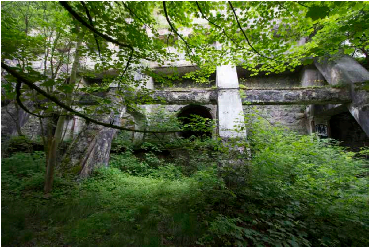
Lime kiln ruin near Buxton, Derbyshire
