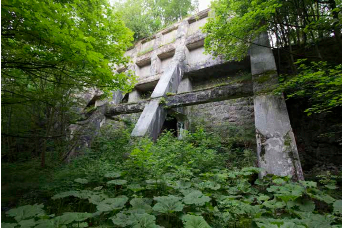
Lime kiln ruin near Buxton, Derbyshire
